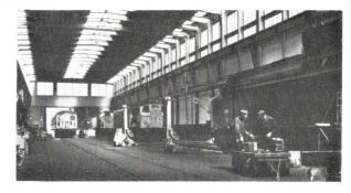
The depot consists of two sheds each having two roads served by inspection pits. The inspection bay roads are wired for testing D.C. locomotives and multiple unit stock. The repair bay is served by a 35 ton overhead travelling crane and is also provided with strengthened concrete strips alongside the track so that locomotive bodies may be lifted using four 20-ton Matterson lifting jacks.
